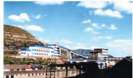
Khutul, "CEMENT-SHOKHO" JSC, Mongolia, 2015
